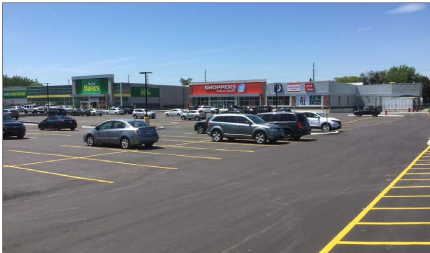
The newly completed Courtice Commons commercial development. Permits for the Food Basics, Shoppers Drug Mart and Dollarama were issued in 2020.
