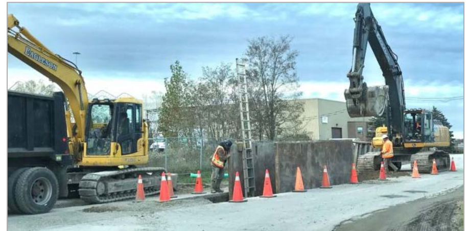
South Courtice servicing construction. 12
