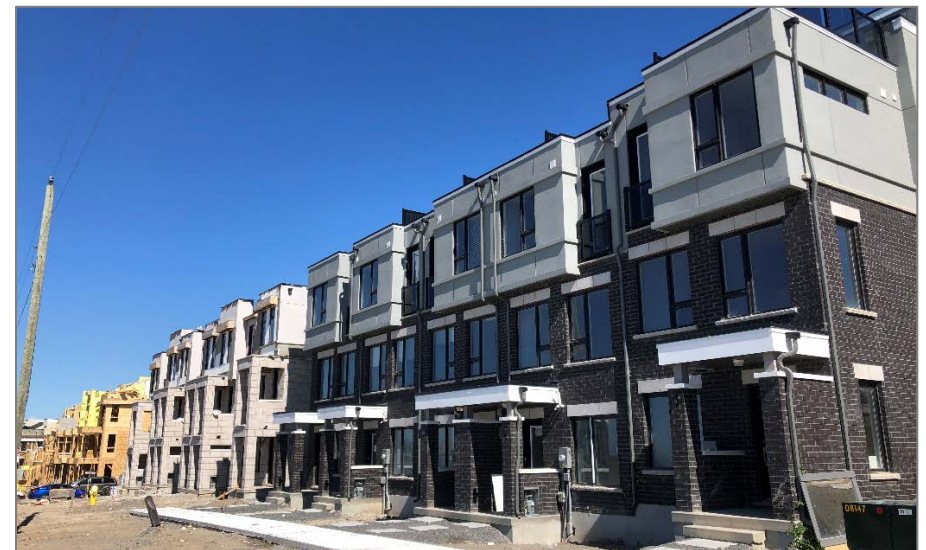
Nearly completed townhouses on Port Darlington Road, Bowmanville.
