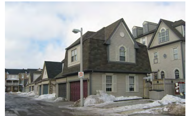
Figure 19. Coach house in a laneway in Oak Park.
