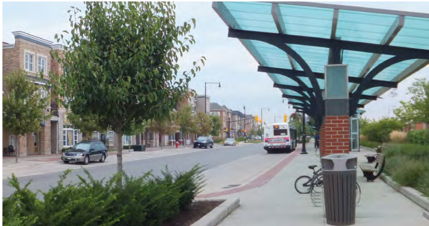
Figure 21. Example of transit oriented development in the Mount Pleasant community (Brampton Sustainable Community Development Guidelines, 2013)
