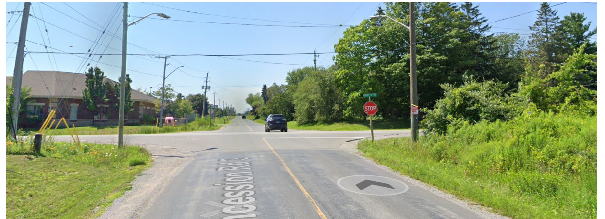
Concession Road 3 looking west at Liberty Street
