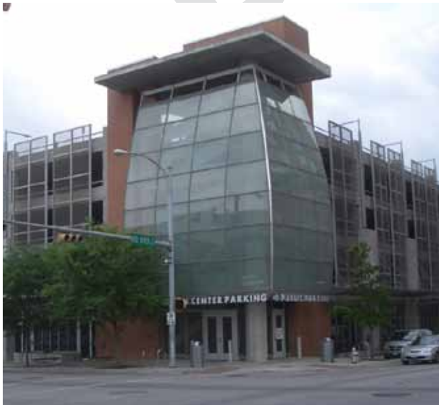
Pedestrian walkway incorporated into parking area.
