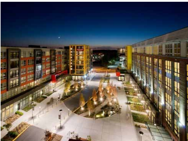
Spanning the Street
