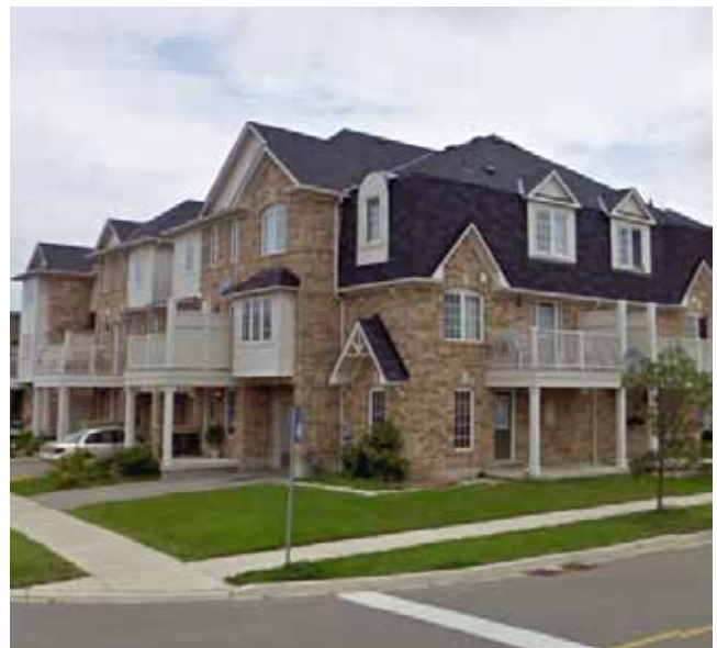
Large building massing is articulated with a variety of techniques including roof forms, entry treatment, dormers and projections
