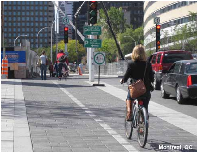
Granite pavers used to distinguish cycle track from sidewalk, Montreal.
