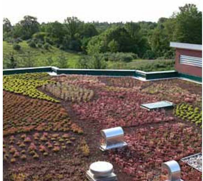
Green roofs are encouraged to achieve a minimum of 80% coverage of the total open roof space.
