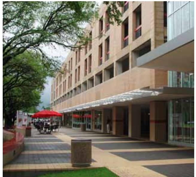
Pedestrian walkway incorporated into parking area.
