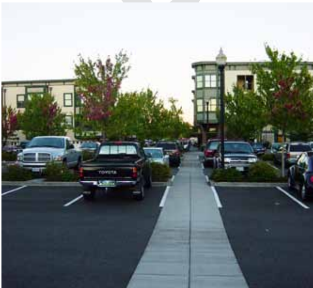
Pedestrian walkway incorporated into parking area.
