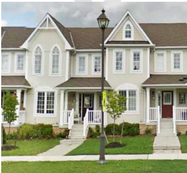
Townhouses with rear laneways are appropriate along arterial roads.
