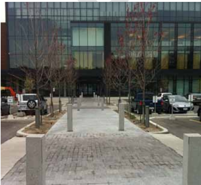
Surface parking with pedestrian walkway and landscaping
