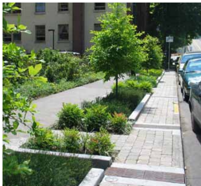
Street tree planting can help manage stormwater run-off by directing water flows into planted areas.
