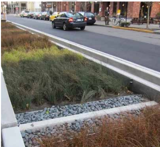
Rainwater harvesting can be used for landscape irrigation reducing unnecessary use of potable water
