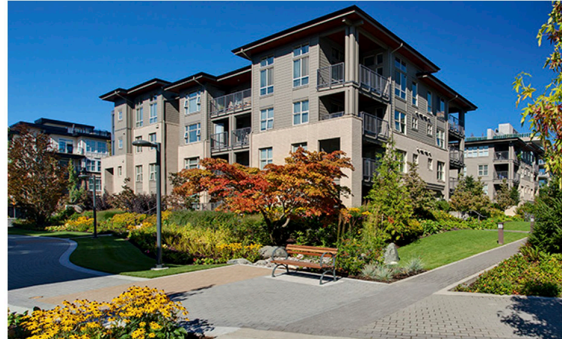
Low rise apartments (Wesbrook Village, Vancouver)
