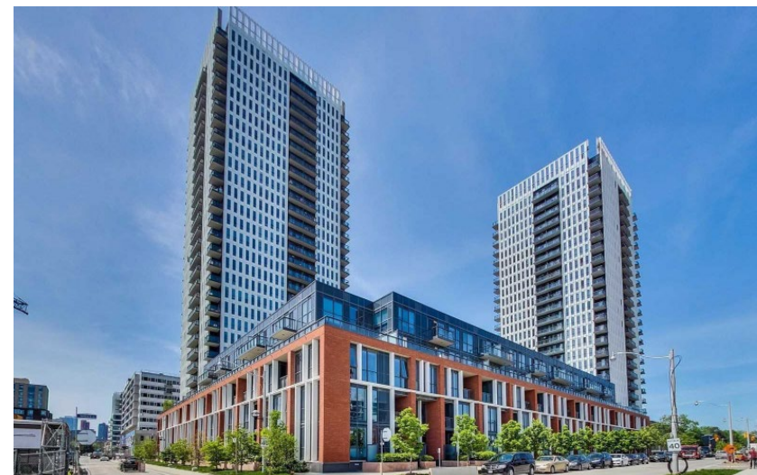
Towers on a low-rise, mixed use podium (Regent Park, Toronto)
