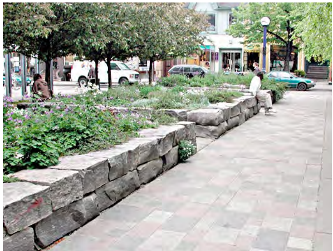
Light coloured pavers assist with the reduction of heat island effect.
