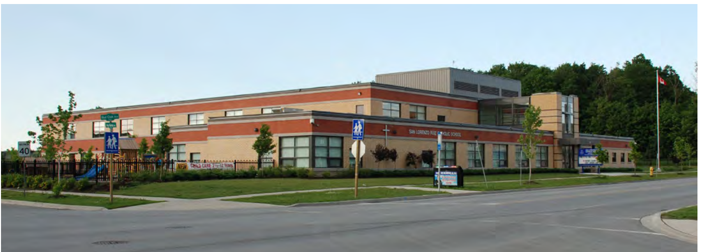
Parking is located to the rear of the building off the main road and the front entrance to the building is directly connected to the public sidewalk.
