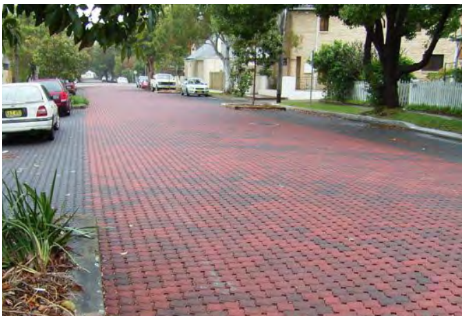
Example of permeable paving material used on a road.
