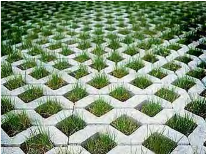
Permeable pavers to support on-site stormwater infiltration.
