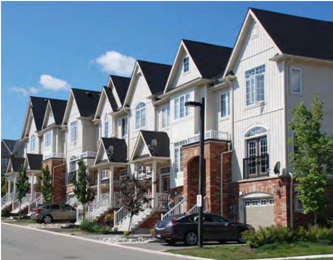
Front garages flush with the front facade.
