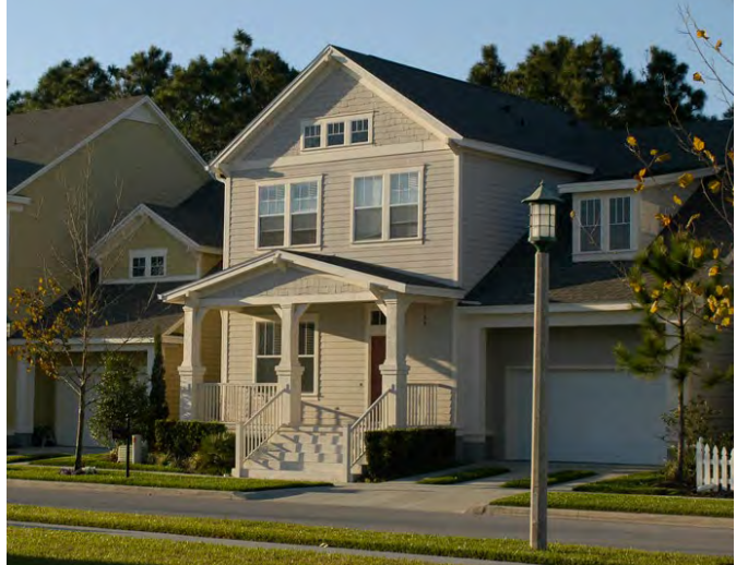
Single detached dwelling with front porch and side garage.
