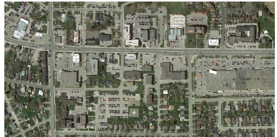
Figure 53. Bowmanville Hospital Aerial View
