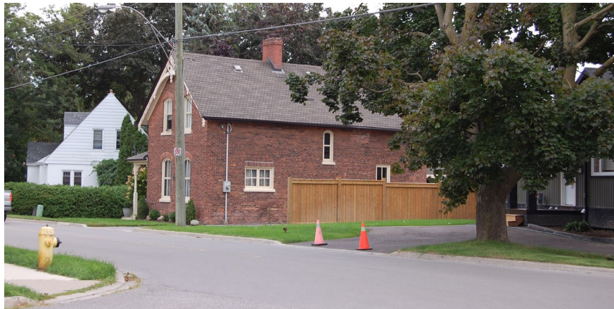
Figure 7. Gaps in the Sidewalk within the Project Area
