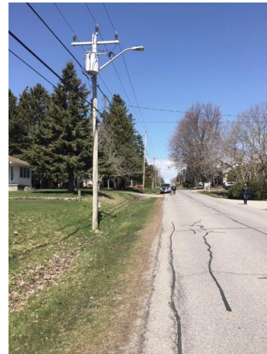
View looking north along North Street
